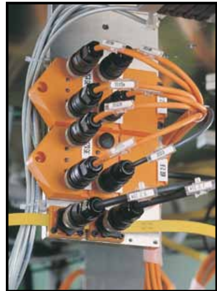
AS-i Module depicted with flat cable and M12 field attachable connectors and junctions.
